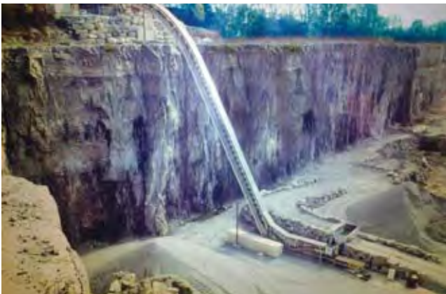
Sandwich belt conveyor for handling 1400 TPH limestone.
