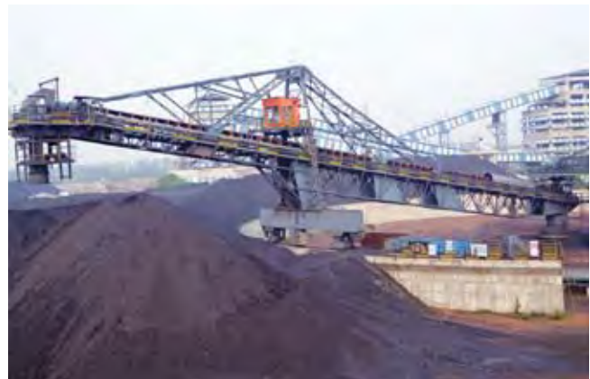
800 TPH radial coal stacker for 70,000 tonne stockpile at IMFA.
